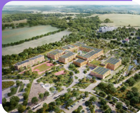
© Jim Clemes Associates S.A.
